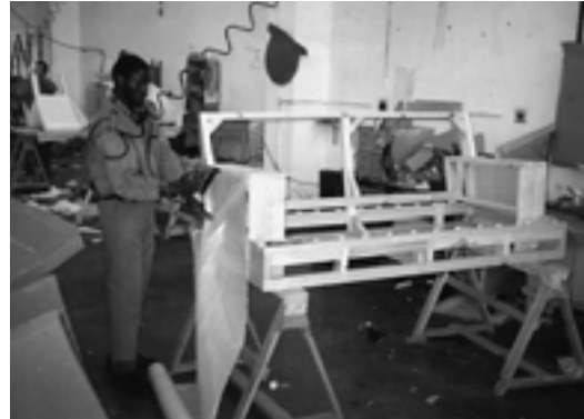
Worker fastening liner to an assembled frame
